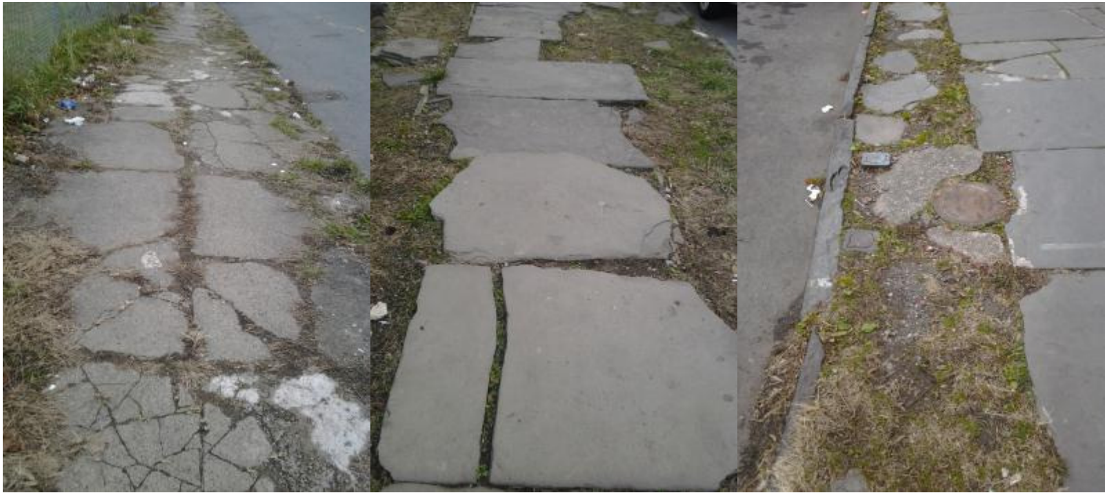
FIGURE 19. SIDEWALK ALONG FIRST BLOCK OF LANDER STREET
